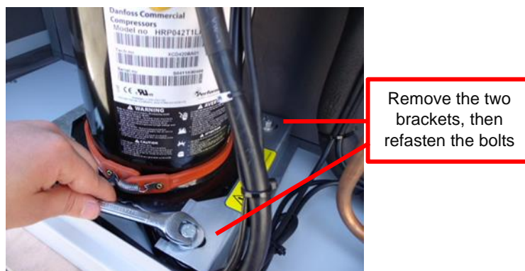
Figure 3-7 Remove Compressor Brackets
