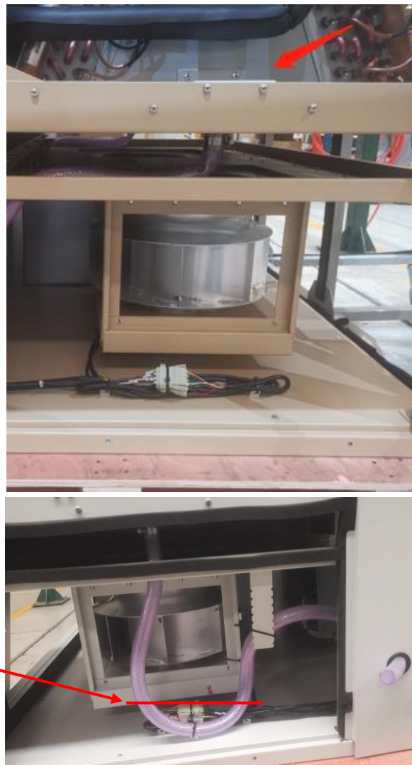
Figure 3-8 Prefill Water to Drain Trap
