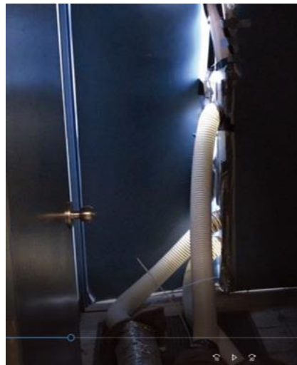
Exhaust air ducting for the IT racks
