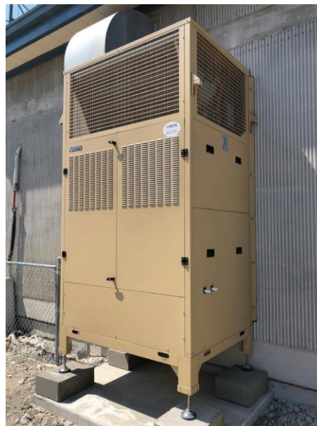
Exterior Shot of Unit 3: AIRSYS UNICOOL Model: 28V1B5MR410BAC
