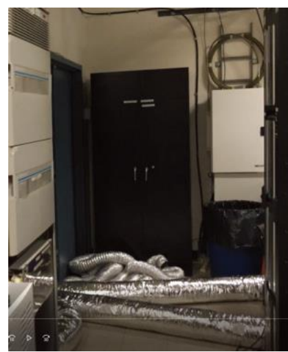
Supply air ducting for the IT racks
