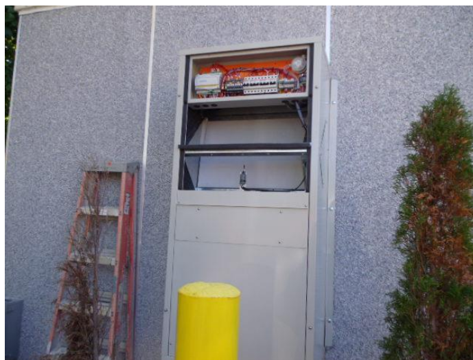
Figure 8: Verify the Unit is Level
