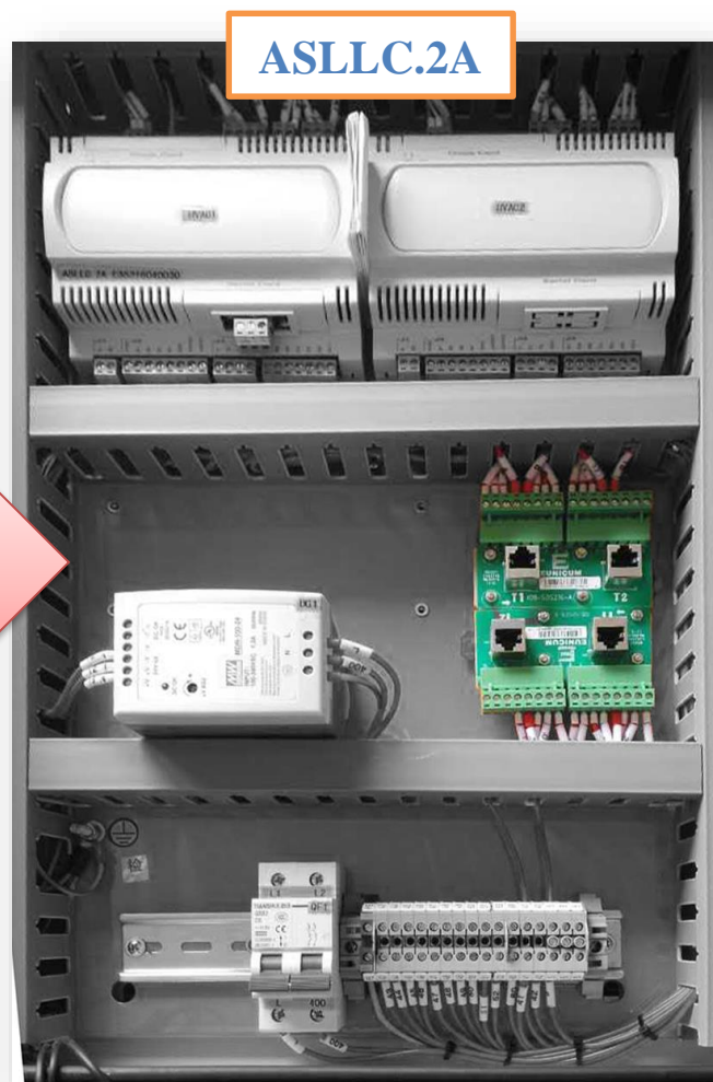
Image 2: ASLLC.2A: Two Cat-5 cable connectors per WPU simplifying field installation of WPUs and ASLLCs
